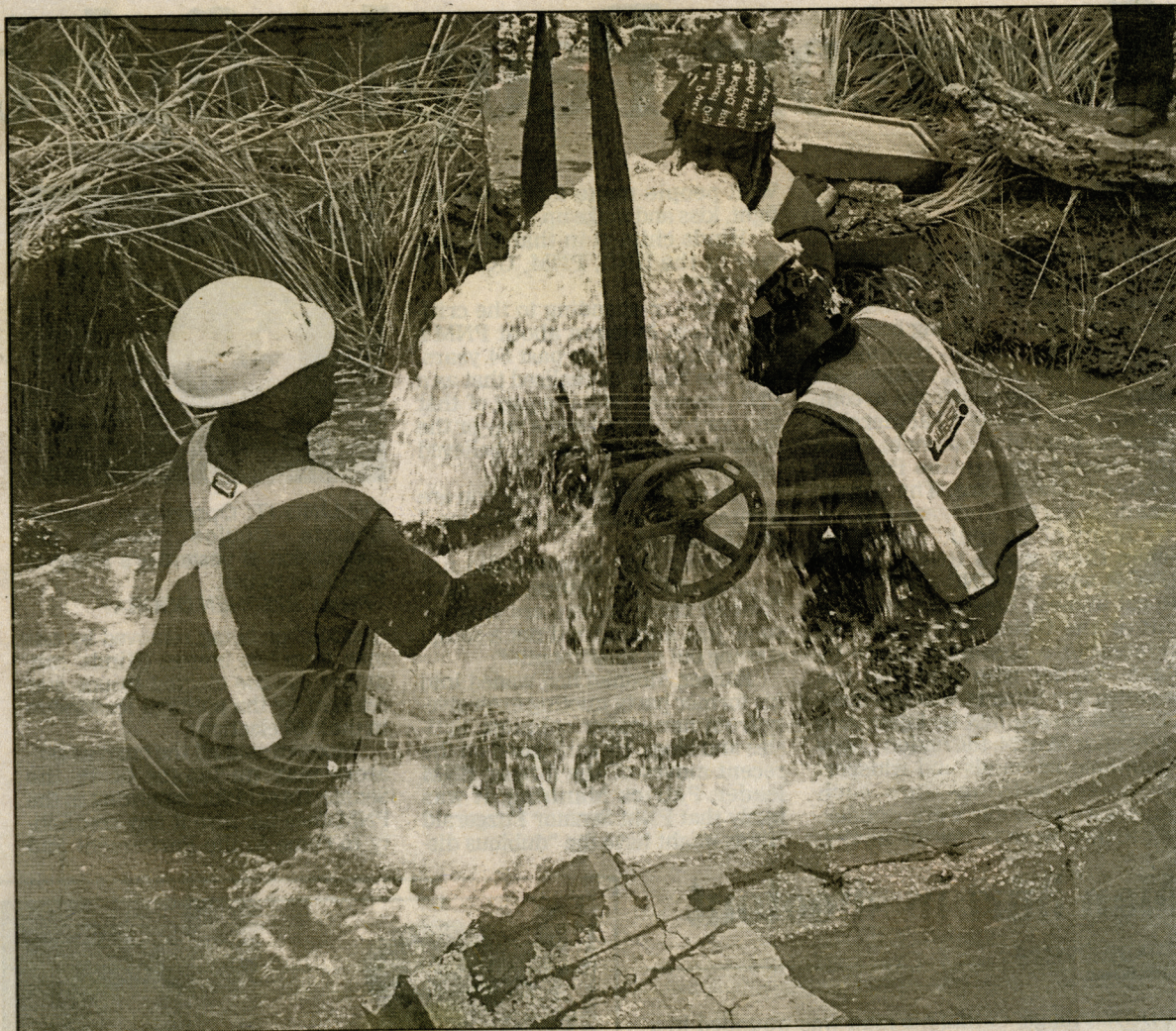
DEEP TROUBLE: WASA pipeline maintenance crew members work in waist-high water to replace the stolen air valve from the 54-inch Caroni South Transmission main near Perseverance in Chaguanas yesterday. —Photo courtesy WASA
